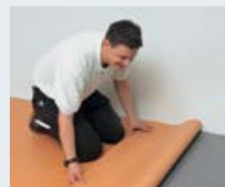
4. Lay in new flooring and press down avoiding stress or distortion
