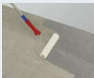
1. Apply special Primer Planus on the subfloor
