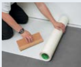
2. Bond Sigan 1 on the prepared subfloor
