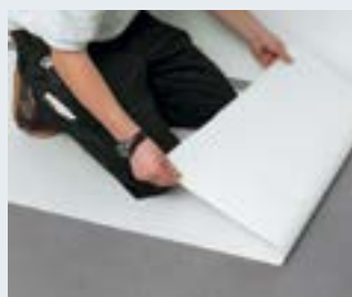
3. Peel the protective paper from the Sigan 1 keeping it flat and straight
