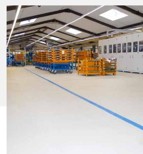
Textured coating KLB-SYSTEM EPOXID EP 236 Screed CT-C35-F5 or concrete C20/25
