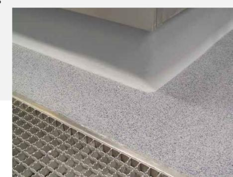
2-c epoxy resin matt sealer KLB-SYSTEM EPOXID -EP 860 or KLB-SYSTEM EPOXID EP 860 Clean
