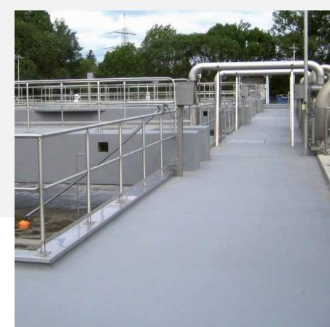
Highly electrically conductive primary layer KLB-SYSTEM EPOXID EP 799 Ableitgrund with a copper band grounding
